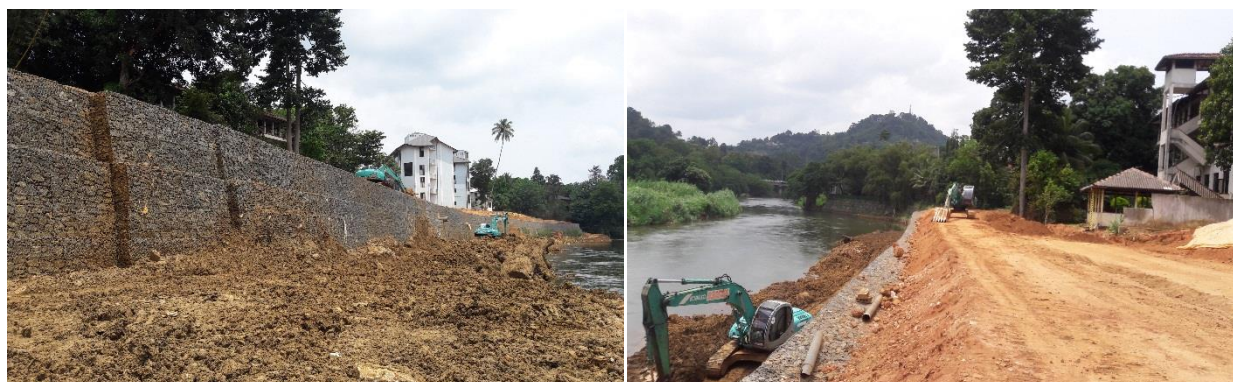
Construction of gabion wall
