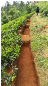
Mechanical Soil Construction – Small drains (Perawatha East Division)
