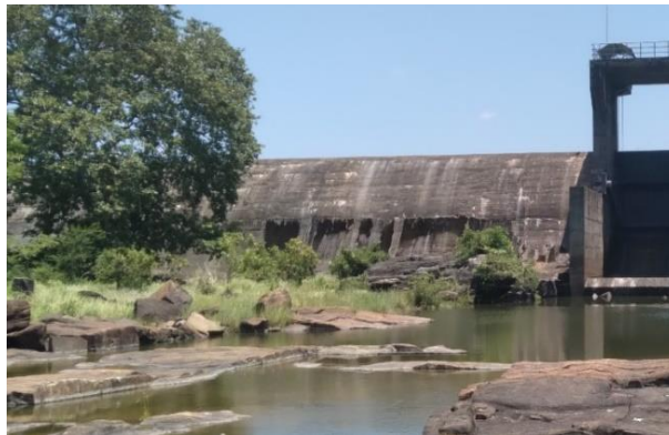
Figure 6 Downstream surface of the Kalawewa natural spillway with the horizontal seepage line at around 124.7 m MSL
