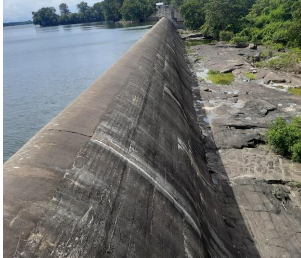
Figure 5 Downstream surface of the Kalawewa natural spillway
